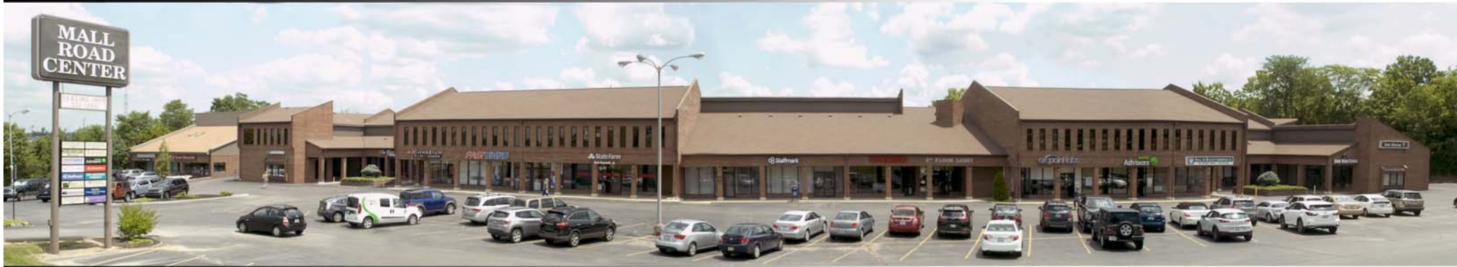
Retail/Office Center in Florence, KY
